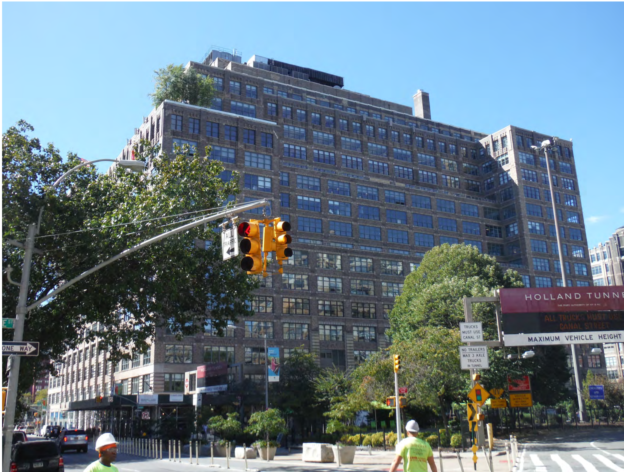
Photo shows very limited visibility of affected windows due to existing pipe rail on parapet
