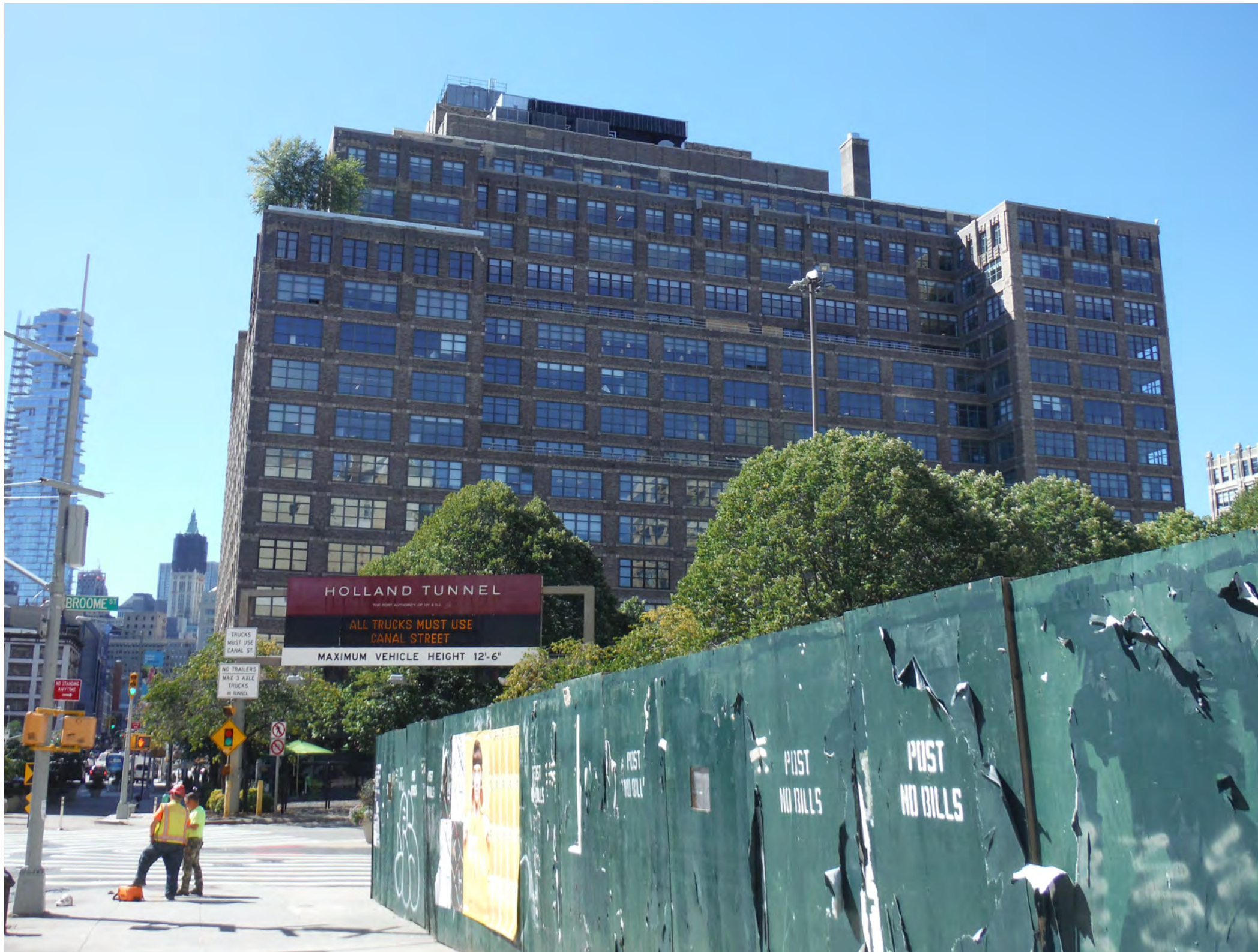
Photo shows partial visibility of affected windows due to existing pipe rail on parapet
